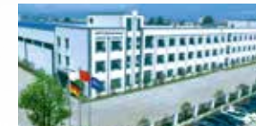
Witzenmann Metal Products (Jiangyin) Co. Ltd. Xiagang Town, Jiangyin City, Jiangsu Province, 214442 www.witzenmann.cn
